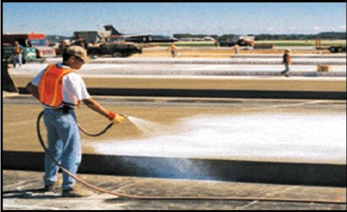
Fig. Wax application process
